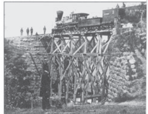
Soldiers of the railroad construction corps could construct such a bridge in a matter of days. From a Mathew Brady photograph.
