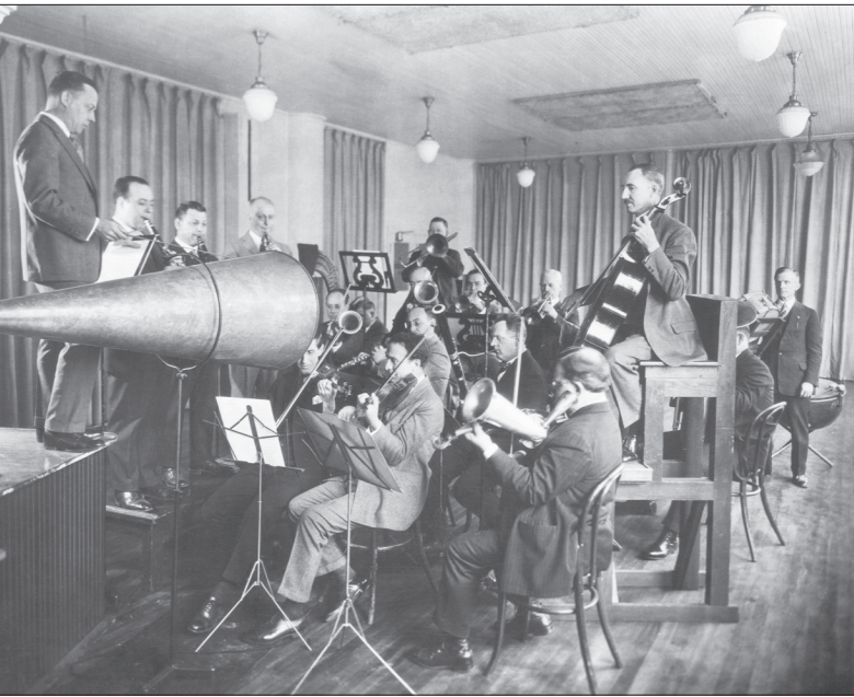
An orchestra makes a recording in this undated photograph. Notice the large recording horn, which was used until the electric microphone appeared in 1925.
