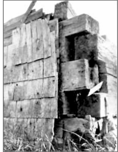
Corner of a house built in about 1690. Note that logs are square and joined by dovetailing, rather than by nails or notches.
