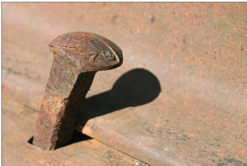
Railroad spike holds the rails in place. Notice the head of the spike is designed to hold the edge of the rail in place as it is secured to the railroad tie.
