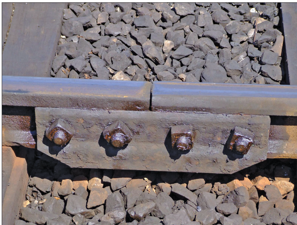
Fishplates are essential to the rails to keep them in place.
