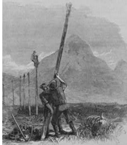
Men installing telegraph poles on the prairie
