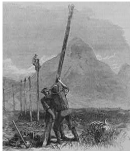
Men installing telegraph poles on the prairie
